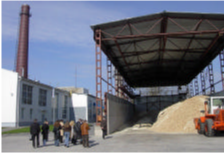
Wood chips storage and boiler house in Daugavgriva
